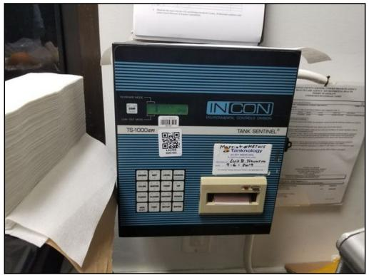
16 : Electronic leak detection system for on-site UST.
